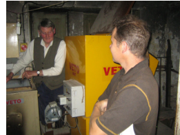
A visitor has the working of the wood chip boiler explained at Acton Scott Hall
