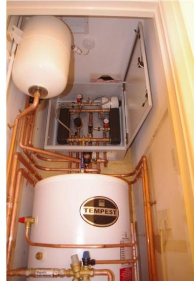
Electrical consumption will certainly be higher, especially in the winter. On sunny days the surplus generation from the p.v. which **goes first** to the house, **next** to the immersion heater, **thirdly** to the electric car charger if required and finally to export may prove enough to keep the hot water topped up most of the time in the superbly insulated hot tank (set at 48 degrees C.)
