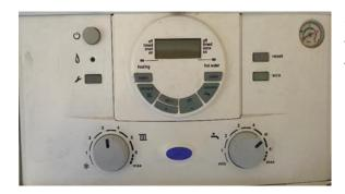
On some boilers there is an "Eco" button which when pressed, stops the pre heating function which uses more gas and just reduces the cold run-off time.
